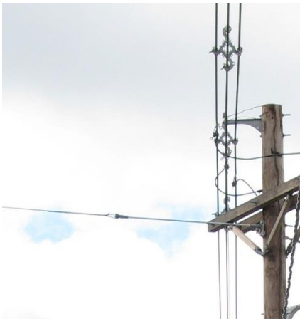
Figure 4.5.12.J Hendrix spacer cable
