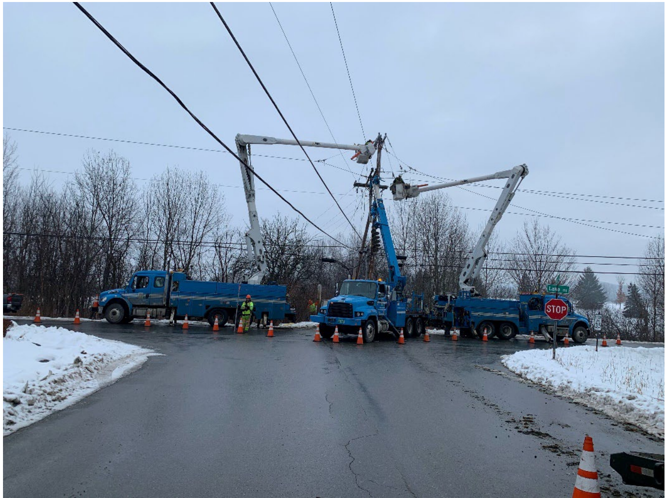
Example of VEC Line Crews repairing a car pole accident.
