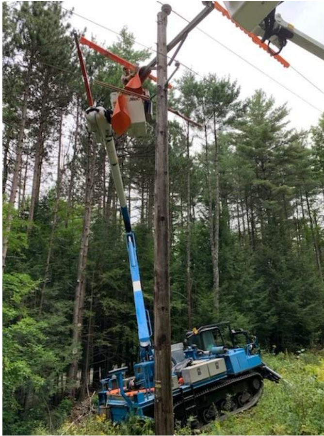
Figure 6.5.3.A VEC Line Crews Utilizing a Tracked Bucket Truck to Access an Off-Road Pole
