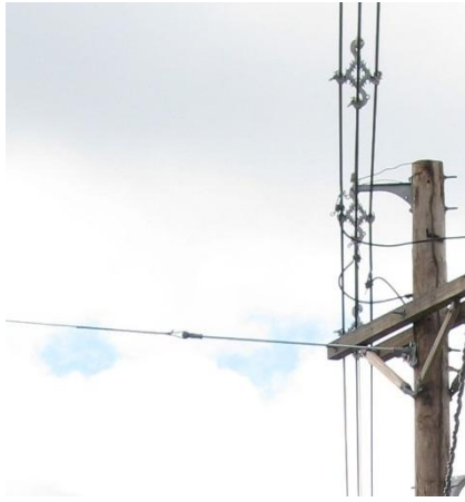
Figure 6.5.3.D Hendrix Spacer Cable
