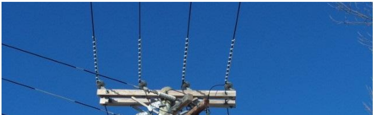
Figure 6.5.3.C Covered Conductor (“Tree Wire”)
