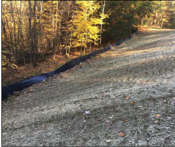
Photo 1: Silt fence correctly installed at the toe of slope along the edge of the work area.
