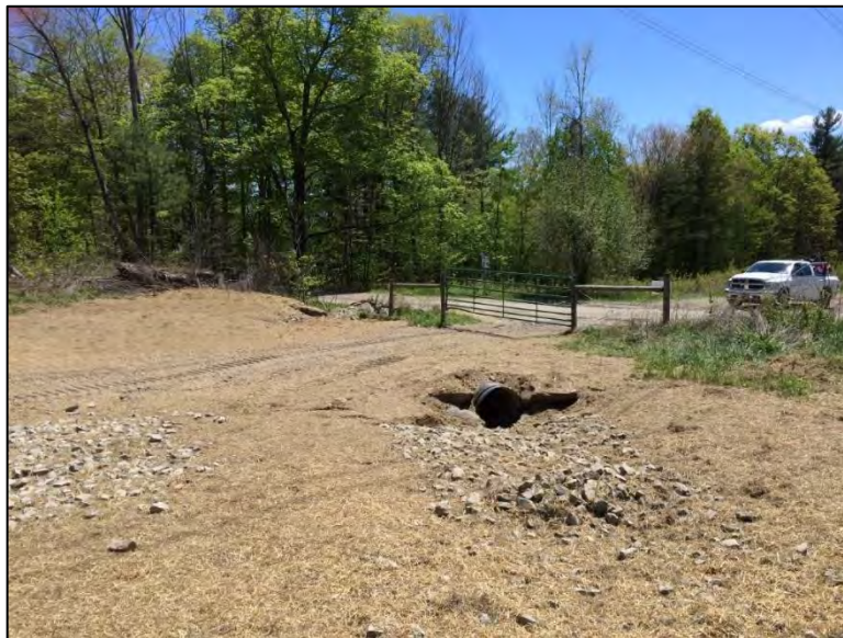
Photo 17: Example of a culvert installed in a non-jurisdictional waterway.
