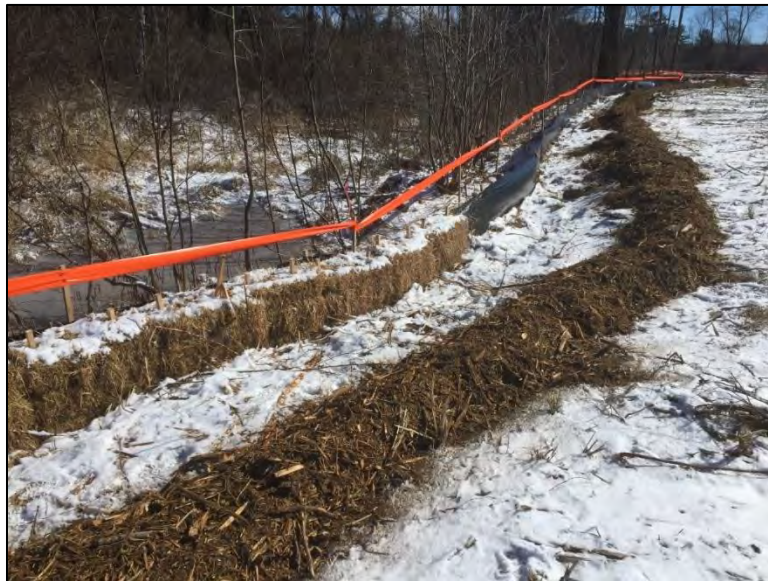
Photo 3: Example of an erosion control mix berm along the edge of a work area. Due to the proximity of resource areas, the silt fence has also been reinforced with a row of haybales.
