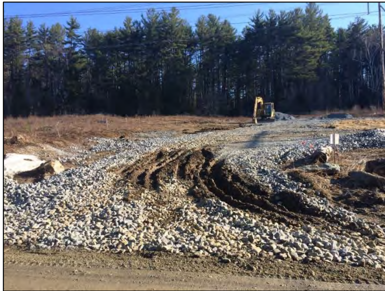
Photo 14: Example of a failed stabilized construction exit. The lack of geotextile below the stone caused the mud below the stone to rise to the surface. After a significant quantity of mud has been trapped by the stone, it must be removed and properly disposed of, and the stone entrance freshened with new material.
