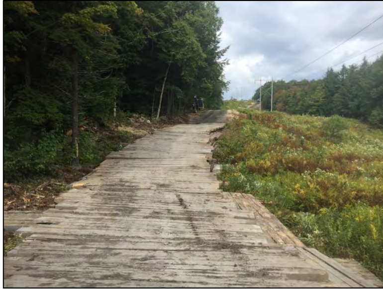
Photo 11: Example of a temporary construction mat access road built out of timber mats. Note that additional timber mats were used on the right-hand side of the photo to raise the grade and create a flat road. Minimal to no earth disturbance was needed to create this access road.
