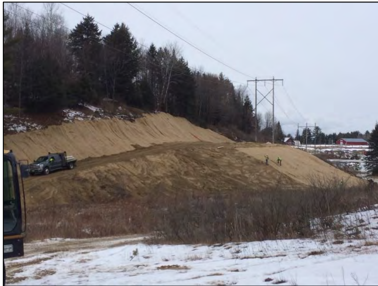
Photo 10: Example of a large cut/fill used to grade in an access road. Note the used of RECP on the steep banks to stabilize the base soil upon final grading.
