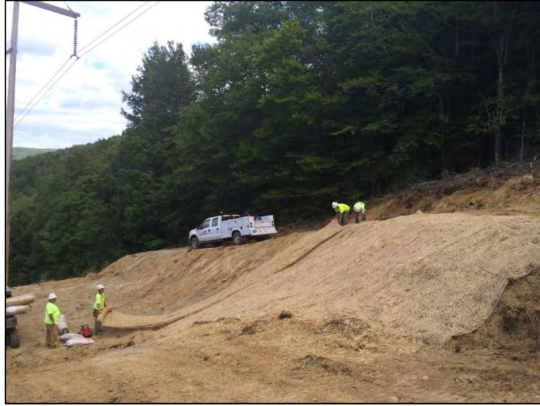
Photo 5: Example of crews installing RECP on a steep slope from an access road shoulder.
