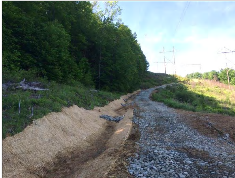
Photo 7: Example of stone check dams installed in a swale stabilized with RECP.
