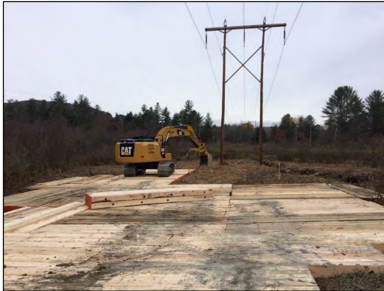
Photo 15: Example of a temporary construction mat equipment pad being installed. Woody vegetation is generally trimmed prior to placement of matting; herbaceous material may simply be flattened as the pads are installed.
