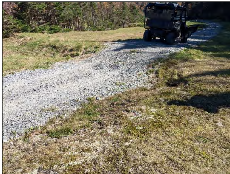
Photo 12: Water bar along steeply sloped segment of gravel work road.
