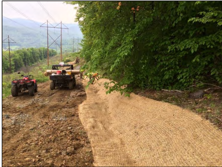
Photo 6: Example of RECP being installed in a swale along an access road.
