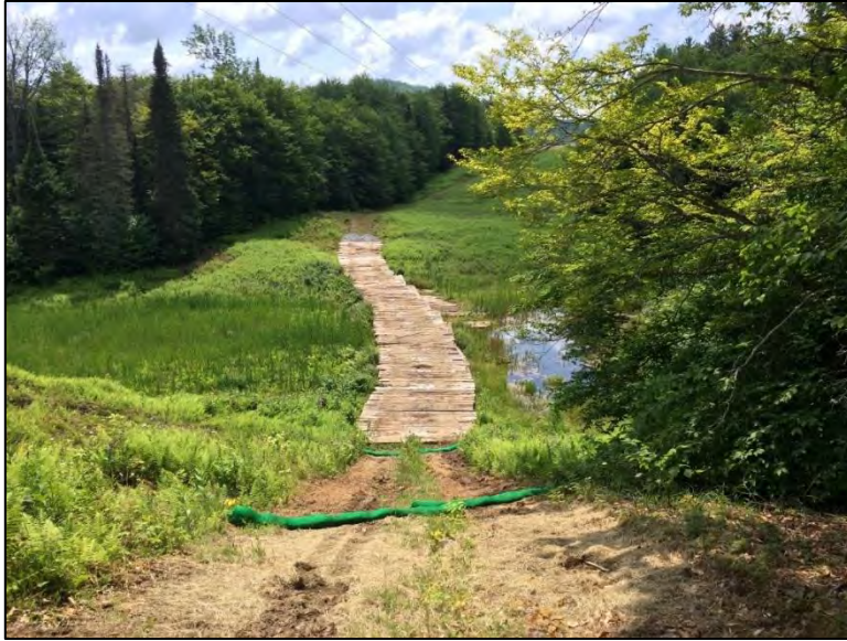
Photo 8: Example of a construction mat road installed through a wetland. Also note the straw wattles used in the foreground to divert water off of the access road (which has been stabilized with seed and mulch) to avoid erosion of the access road into the wetland.
