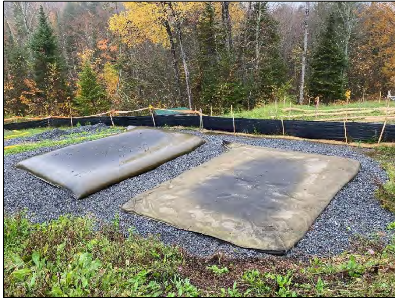
Photo 19: Example of a dewatering filter bag installed on top of a stone bedding.
