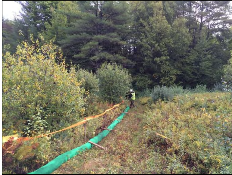
Photo 2: Example of straw wattle being installed prior to any earth disturbance.
