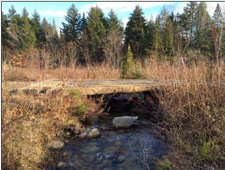
Photo 9: Example of a temporary bridge over a stream built out of timber mats.
