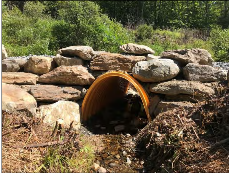
Photo 16: Example of an open bottom arch culvert installed over a perennial stream.
