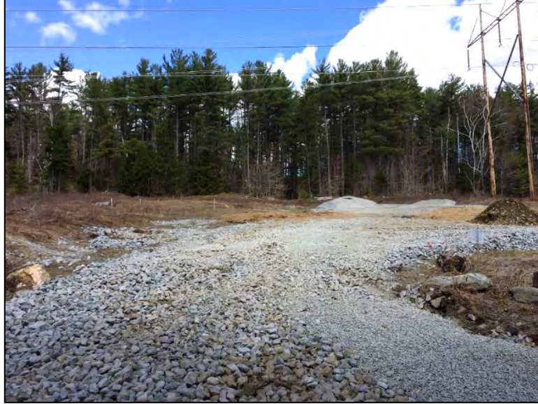
Photo 13: Example of a stabilized construction exit.
