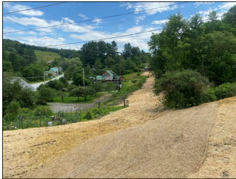
Photo 4: Example of various mulching products used in one area. Hay or straw is used on the flatter areas, while a RECP is used on the steeper slopes (3:1 or greater).
