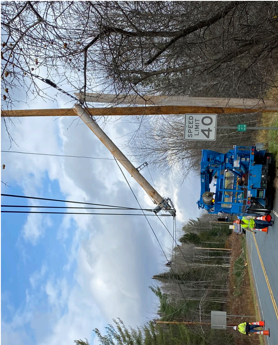
The high winds that swept through Vermont on Halloween snapped this pole on along Route 243 in North Troy. Several other poles in VEC territory were broken during the storm. Here, crews prepare to lift then attach wires to the newly installed pole.
